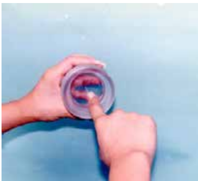
Photo 11 Greasing the Coupling
