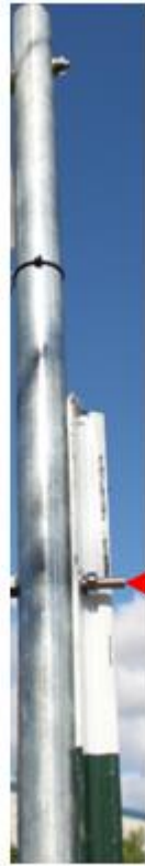
Figure 1: Hurricane Pole and Fence Post Attachment
