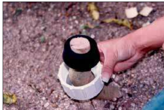
Photo 10 Installing the compression ring
