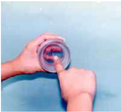
Photo 11 Greasing the Coupling
